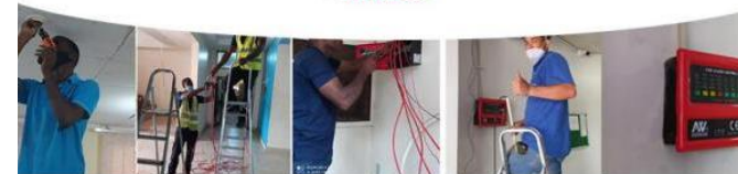
Nigeria ENUGU ElectricityL Distribution Company
