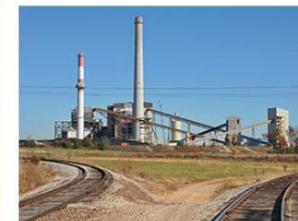
Fired power plant
