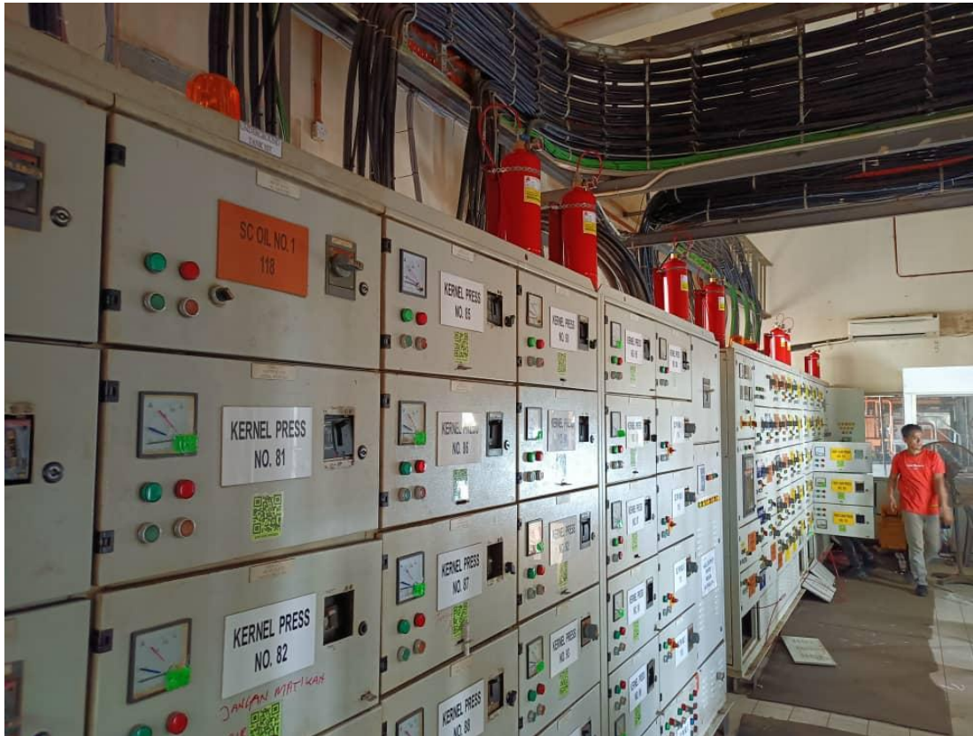
Fire detection tube suppression system
