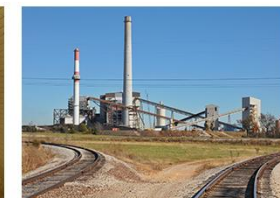
Fired power plant
